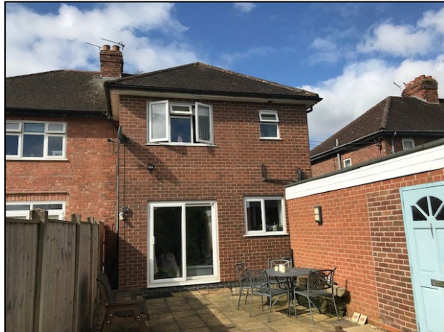
Photograph showing where the proposed single storey rear extension would be located and the existing garage which would be demolished.
