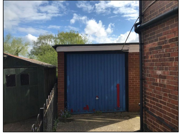
Photograph showing existing garage which is proposed to be demolished to provide space for the proposed single storey rear extension.
