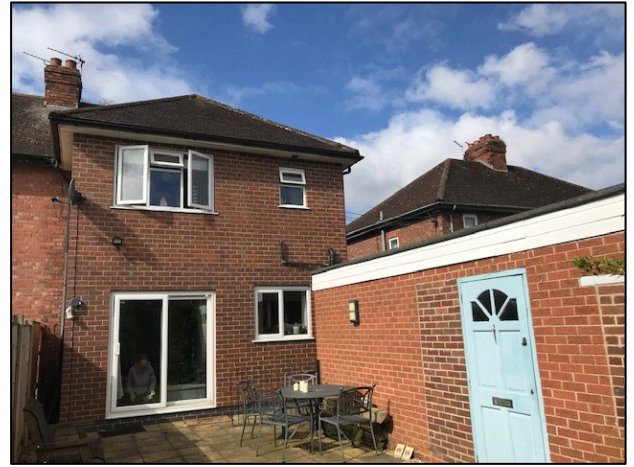
Another photograph showing where the proposed single storey rear extension would be located and the existing garage which would be demolished.
